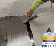
Poly Fix<sup>®</sup> is can also be used as concrete repair binder to repair hair line cracks or mixed with dry sand to patch/repair concrete spalls, pop-outs, or control joints.
