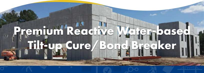
A chemically reactive water based tilt-up cure/bondbreaker specially engineered to provide a clean, easy lift of tilt-up panels and meet the moisture retention of ASTM C 309. SpecTilt WB contains no diesel, kerosene, waxes or silicones.
