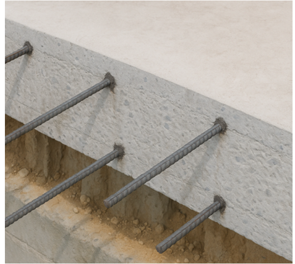
Rebar Foundation Extension
