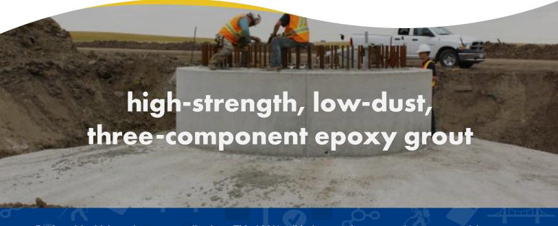
Designed for high-performance applications. This 100% solids, low-exotherm grout features a special aggregate blend that ensures excellent flow and uniform distribution throughout the epoxy matrix. SpecPoxy Grout LD is ideal for deep pour applications, offering long work time and superior bonding for installations requiring high compressive, bond, and tensile strength.
